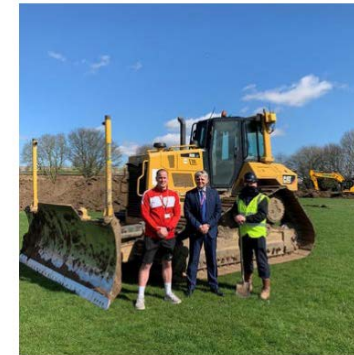
Groundworks commence at Haven High Academy for the 3G pitch
